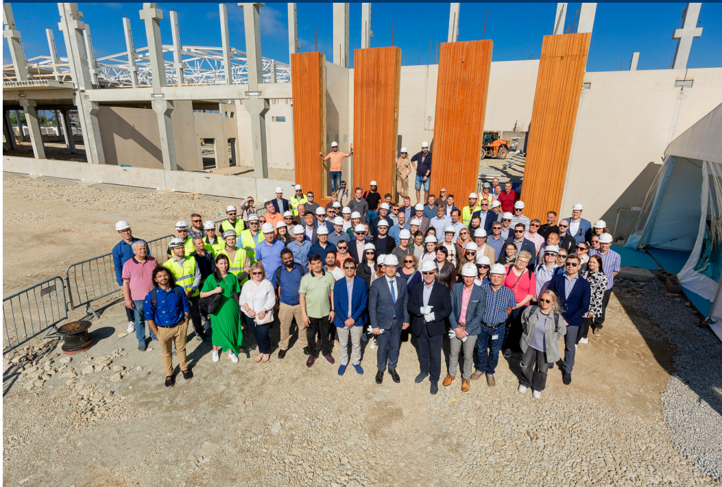
Development of a new 360 MW production facility. Tallinn
