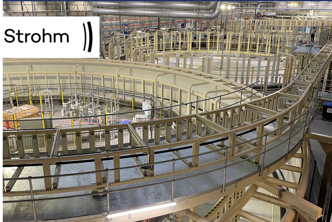
Strohm's TCP pipeline plant in Ijmuiden, Port of Amsterdam
